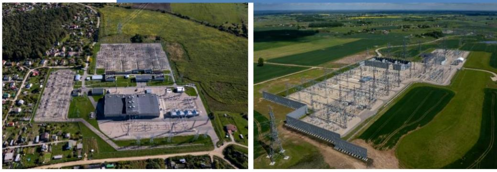
Electrical and gas connections
